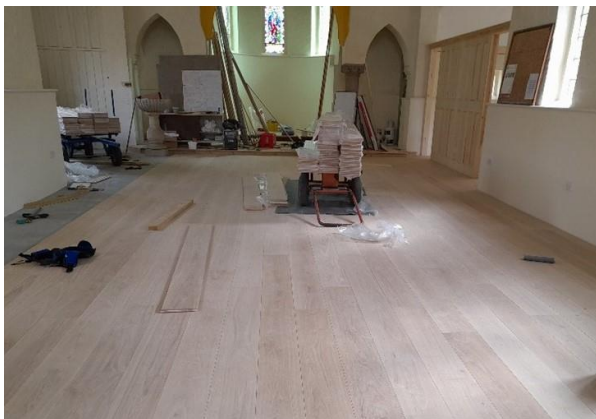
Nave – looking East
